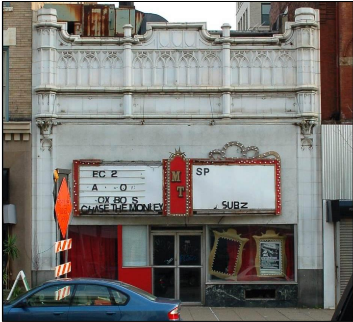
Photo: Justin Greenawalt 6018 Penn Avenue, Prior to Demolition, 2014
