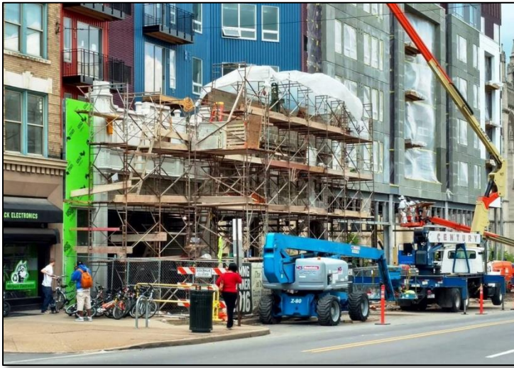
Photo: Justin Greenawalt Reinstallation of 6012–6014 and 6018 Penn Avenue Facades, May 2016
