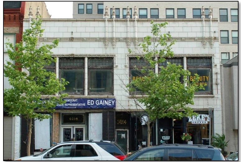
Photo: Justin Greenawalt 6012–6014 Penn Avenue, Prior to Demolition, 2014
